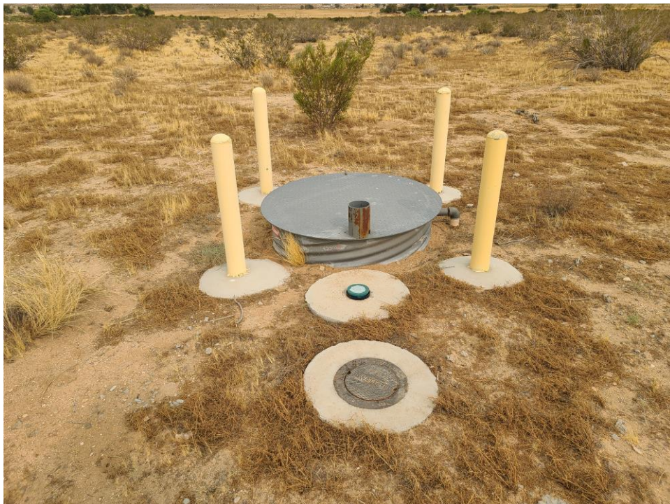
Looking at Mojave Water Agency Water Line Easement along Helendale Road
