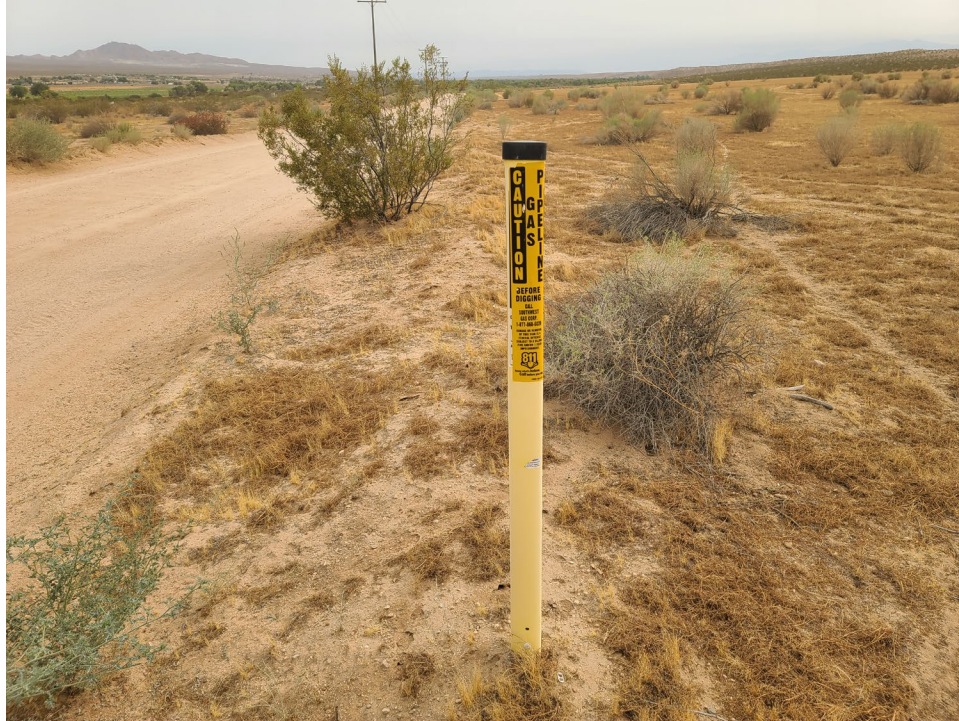
Looking Southerly at Natural Gas Line along Helendale Road
