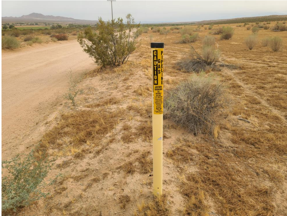
Looking at Natural Gas Line along Helendale Road
