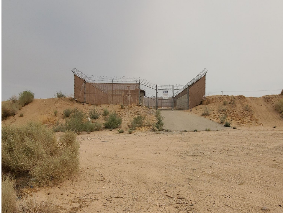
Well Site #26081 along Helendale Road and west property line
