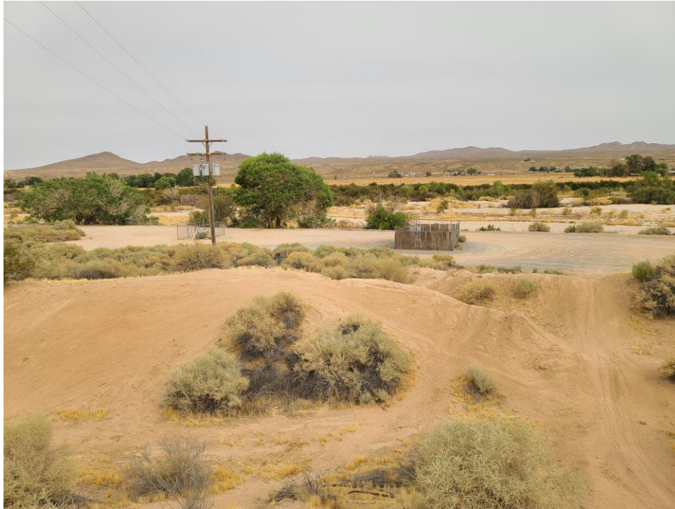
Looking at well sites and power poles near Mojave River
